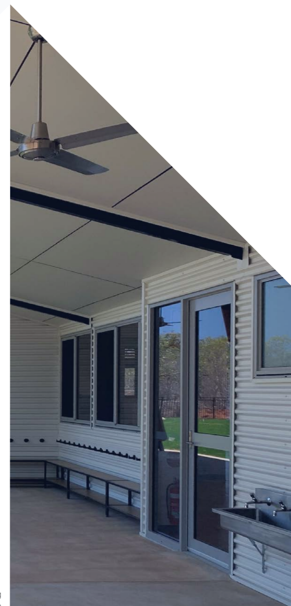
St Mary's Pre-Primary Building H&M Tracey Construction
