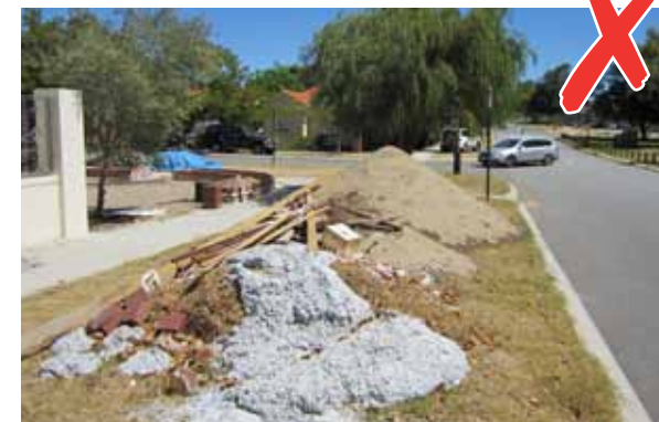
Sand and concrete stockpiled outside of construction site.
