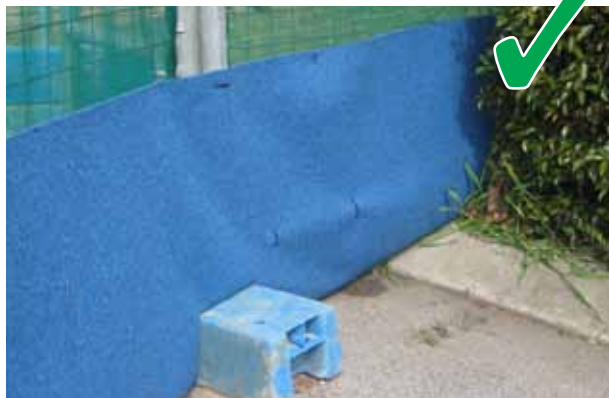
Sediment control fencing abutting vegetation prior to earthworks.
