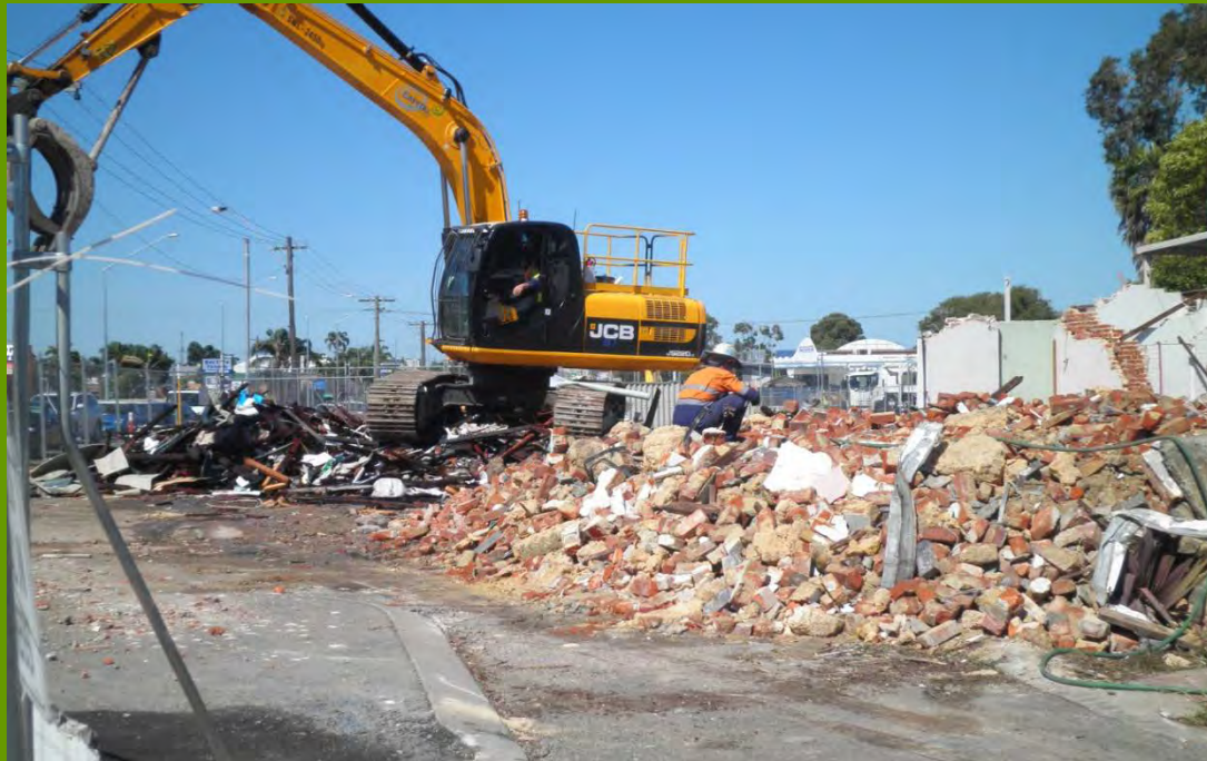
Demolition site for Gateway Project, Belmont
